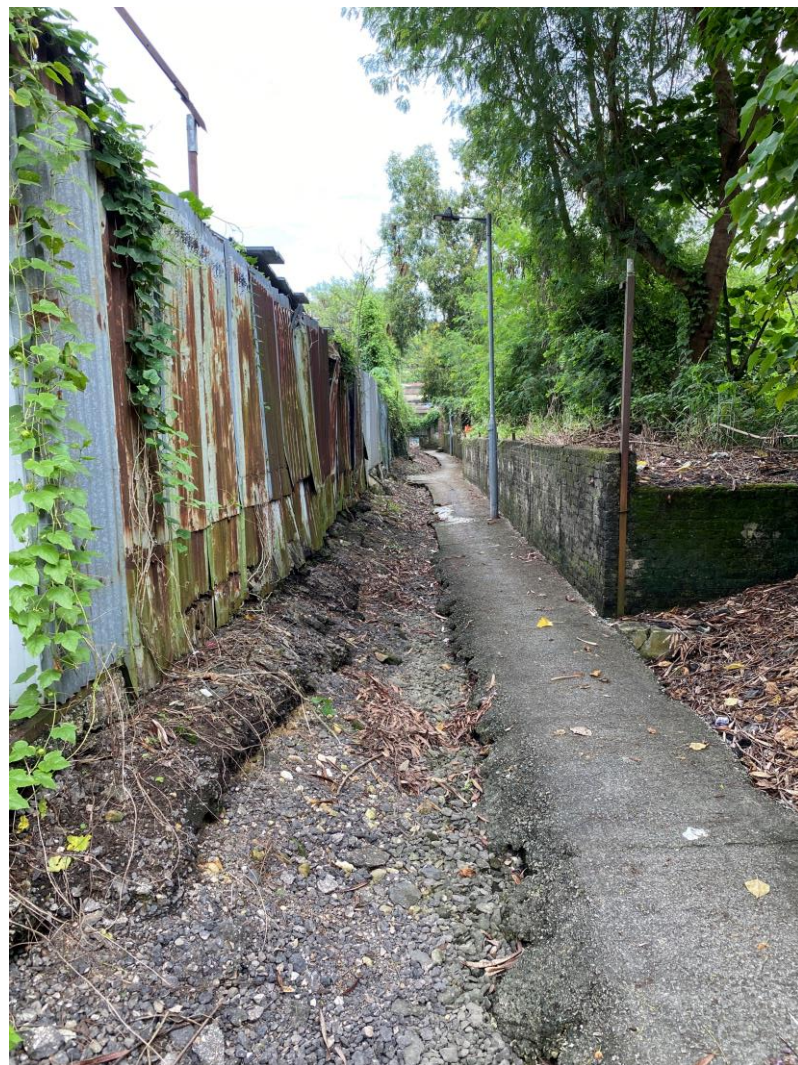
Photo 1: Footpath at east of the Project Site
